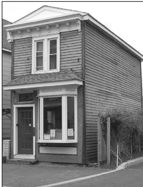
Above: Facade improvements are underway at 19 N.W. Front Street.
